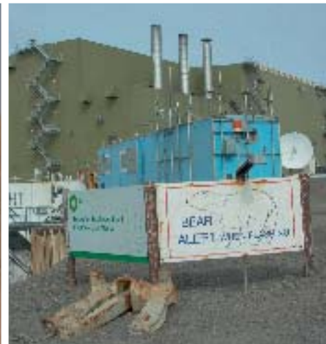
The 26,000-ton, 610-foot-long plant was designed to treat 2 million barrels of seawater daily, for injection into the Prudhoe Bay reservoir to maintain pressure and enhance production
