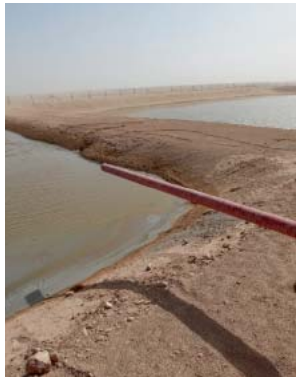
Water for drilling mud, Oman
