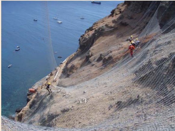
Installation of rockfall containment netting, St Helena
