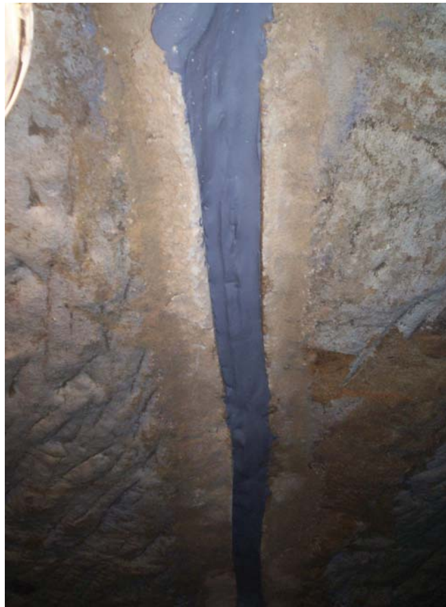
Figure 8: The width of the sealant is approximately 70mm
