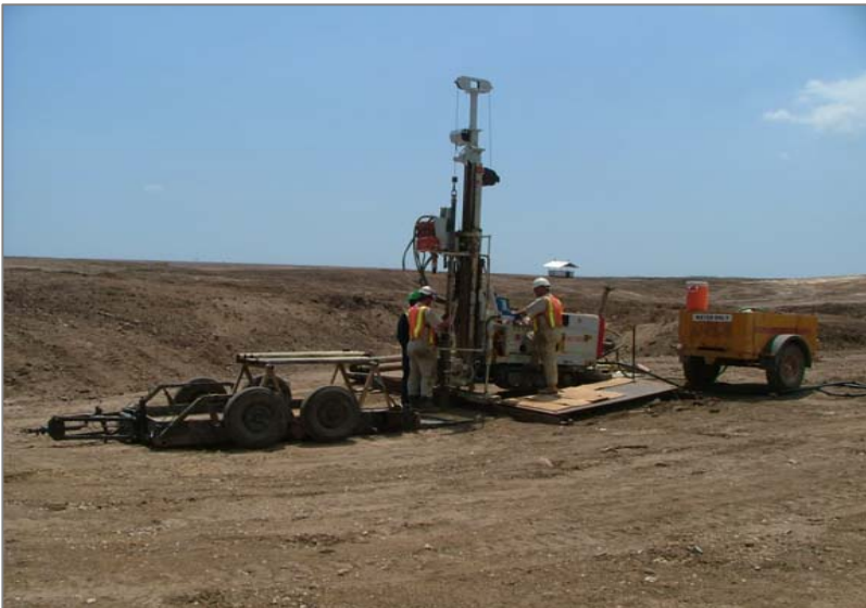
Photograph showing EMD rig undertaking Geotechnical investigations for voids. Caribbean 2006
